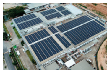
Solar panels installed at HOYA LAMPHUN LTD. (annual generating capacity: 2,200 MWh; reduction in annual CO 2 emissions: about 1,000 t-CO 2 )
